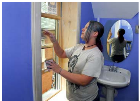
Robert Wilson/Record staff Painter Julia Skinner sands down the washroom window casings.
