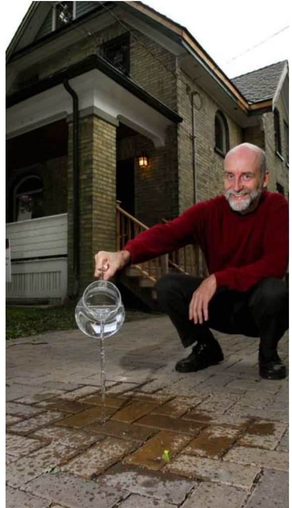
Robert Wilson/Record staff Ben Barclay, project manager, demonstrates how water will soak into the eco-friendly engineered driveway.
