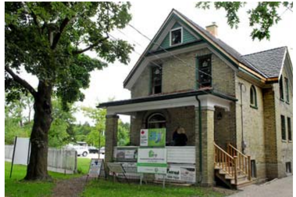
Robert Wilson/Record staff REEP has retrofitted and renovated this century-old Kitchener house at 20 Mill St. with every conceivable green idea.
